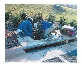
After removal of mulch and debris, measure distance from the top of the
